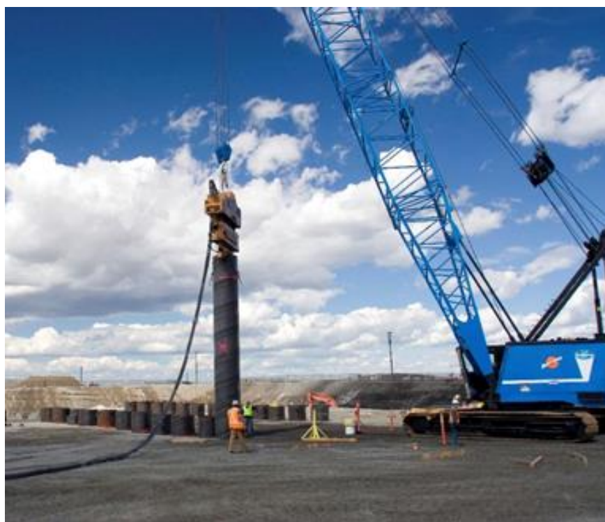
Exhibit V- 6a: Over-Casing Being Driving into the VPUs (Charboneau, 2015)
