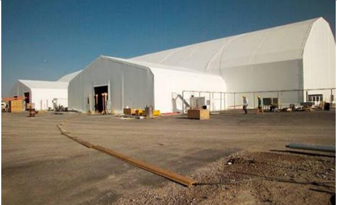
Exhibit IV- 1: Typical Environmental Enclosure Used at INL
