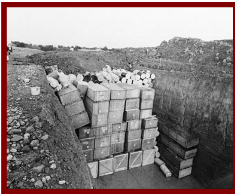
Exhibit II-3: SDA Waste Disposal - Open Trench Photo
