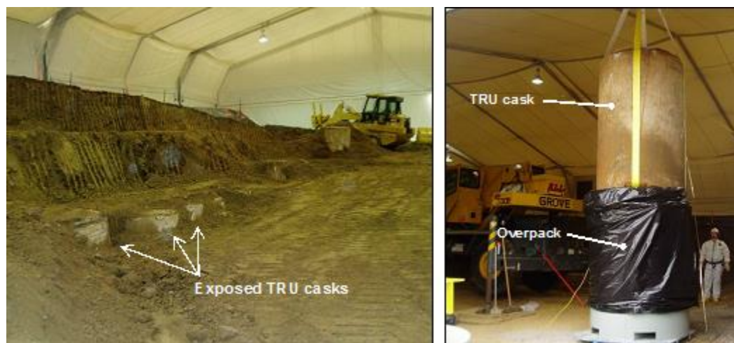
Exhibit IV- 6: Interior of Enclosure Showing TRU Casks and Cask Transfer
